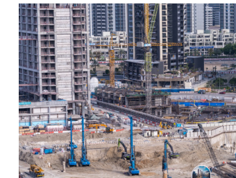
HIGH-RISE BUILDING CONSTRUCTION
