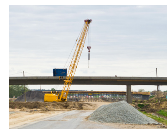
ROAD AND HIGHWAY CONSTRUCTION
